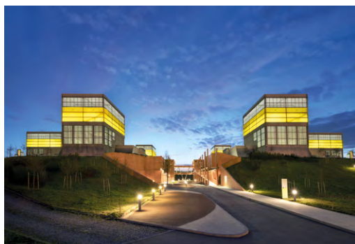
Green Data Center ENI
